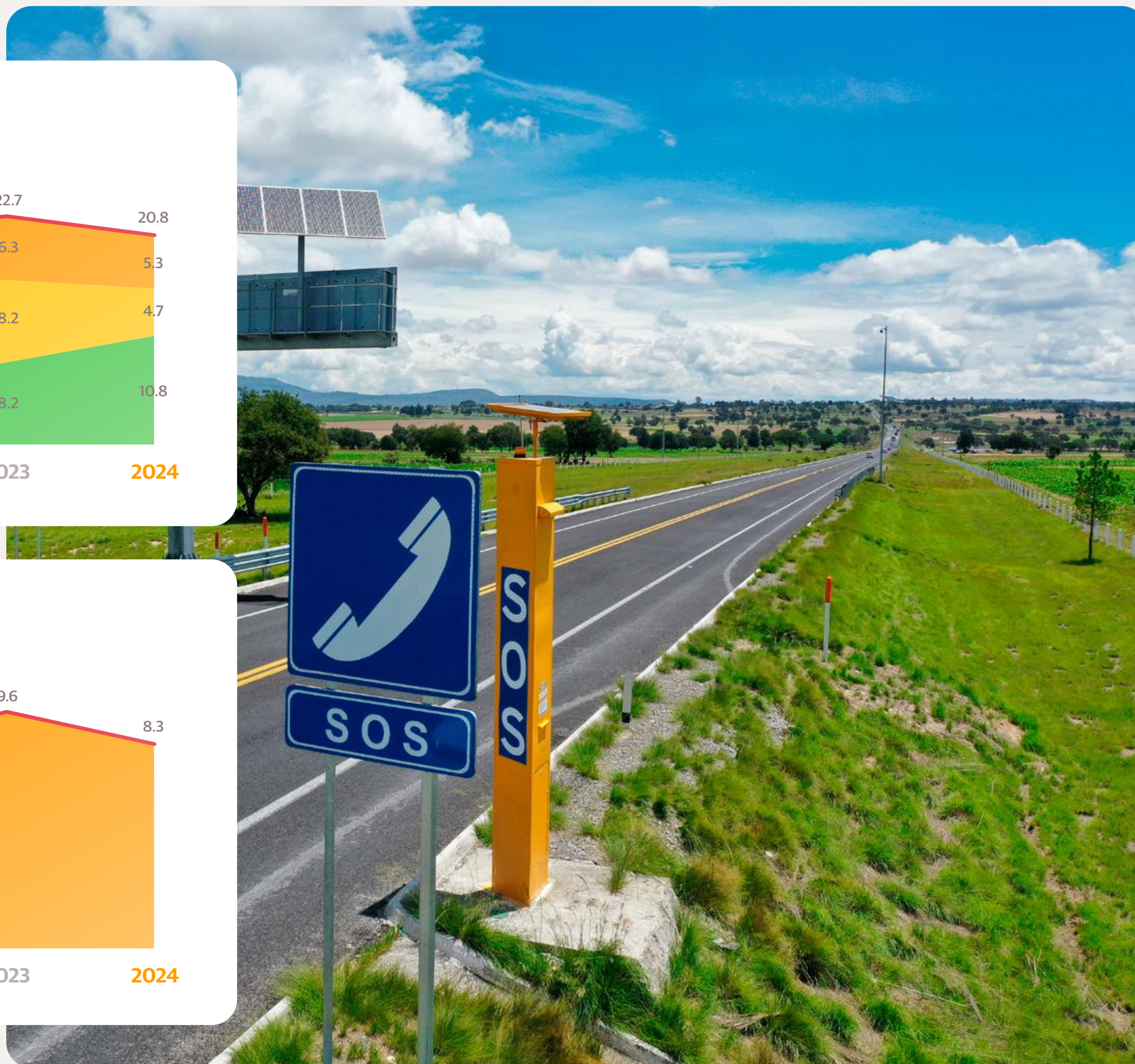
Autopista Amozoc-Perote, Mexico
